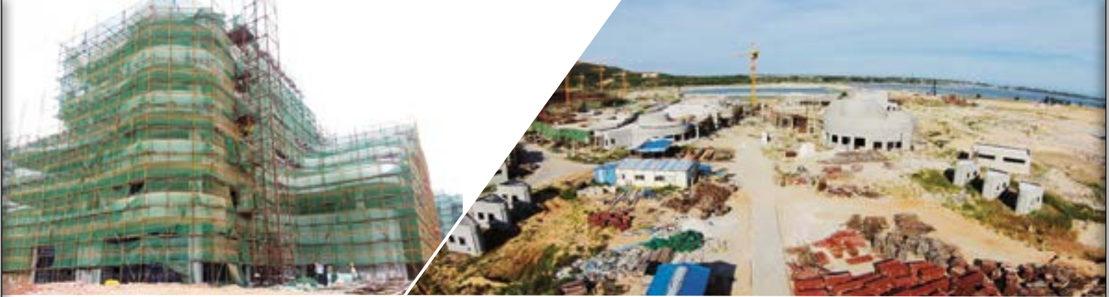
IMAGES: Ocean Paradise, Hainan Island, China under construction
