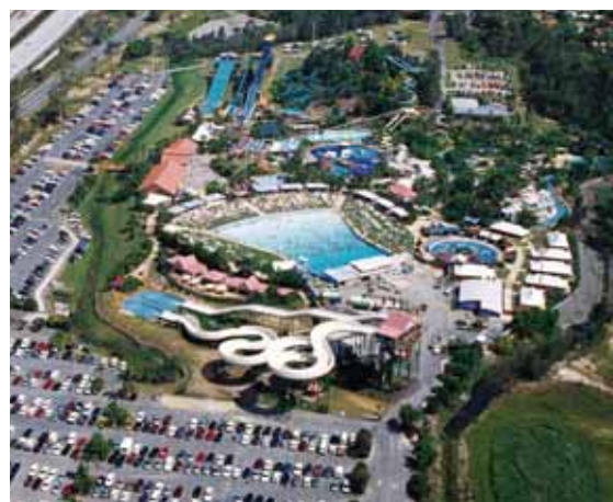
Aerial view of Wet 'n' Wild Water World, Gold Coast, Queensland. ↑
